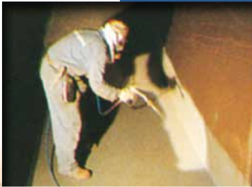
After blast cleaning to Sa 2½, apply Chemflake Special
