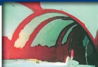
Studsrup Power Plant
